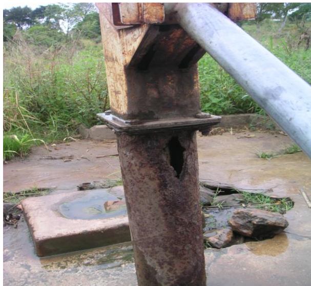
Figure 2: Borehole metal corrosion that could be due to chloride concentration in groundwater
